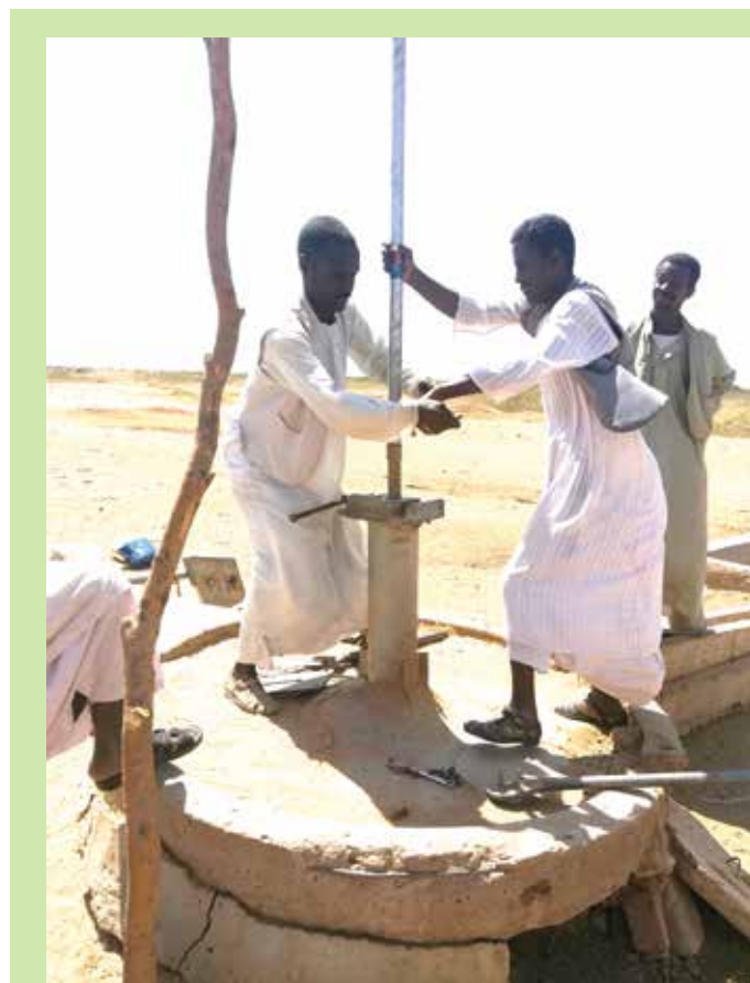
Returnee community from Darrasta repairing hand pump after receiving tools and training from Aqua4Sudan
